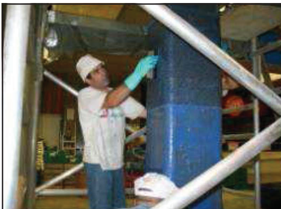
Application of Saturant on FRP Wrapping
