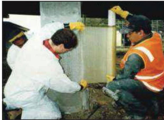
Wrapping with Glass Fiber
