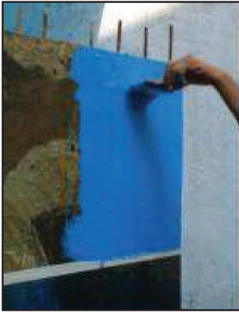
Application of Saturant
