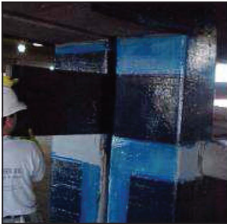
Wrapping with Carbon Fiber
