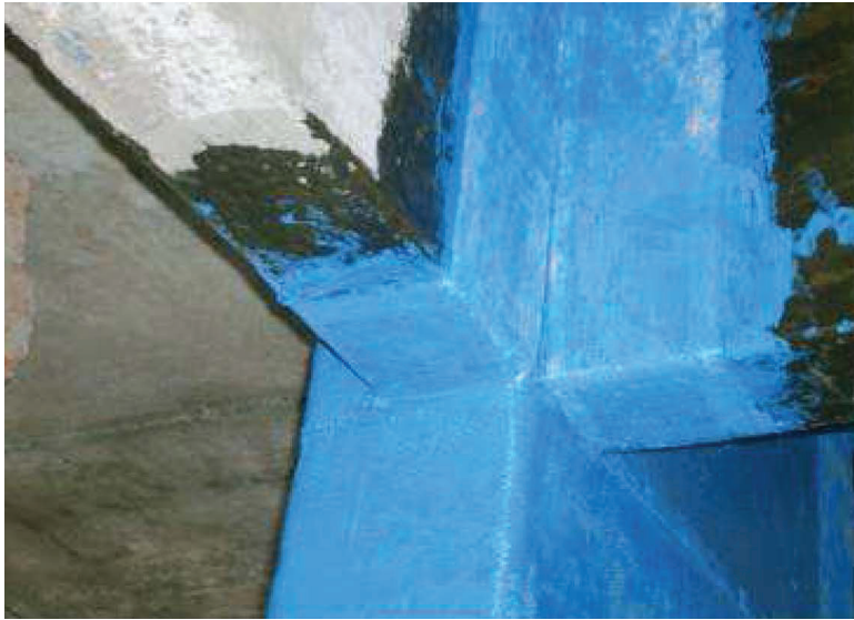
RC Columns after Completion of FRP Wrapping
