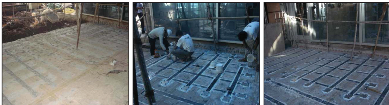
Fig 18 Strengthening of slab from above using Carbon Fibre Composite laminate with anchor plates at the end
