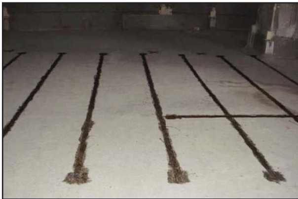
Fig 20 Strengthening with Carbon Fibre Laminate system.
