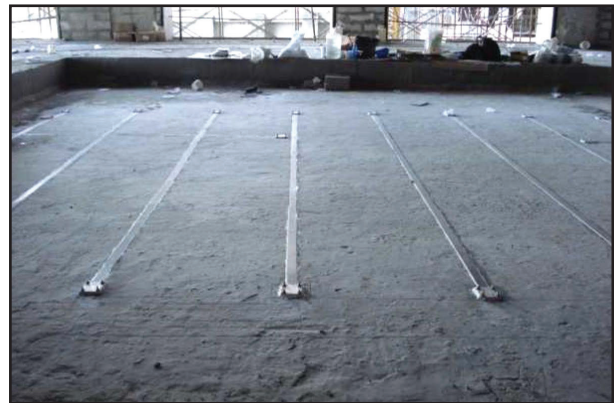
Fig 20 Strengthening with Carbon Fibre Laminate system.
