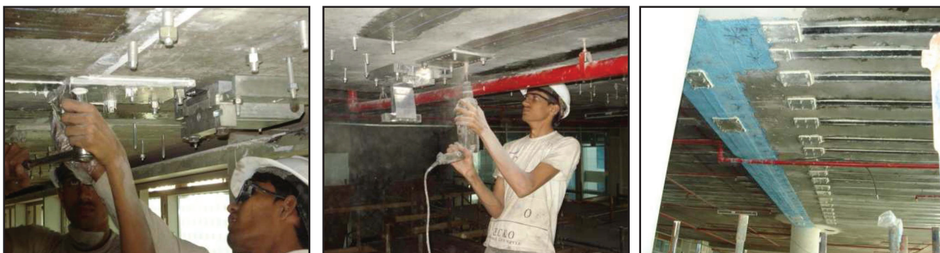
Fig 19 Strengthening of slab from below using the Pre-Stressed Carbon Fibre Laminates With anchor plates at the end
