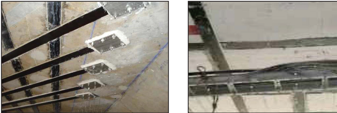
Fig 5 Use of Laminates in for strengthening of slabs in a bridge and a building.
