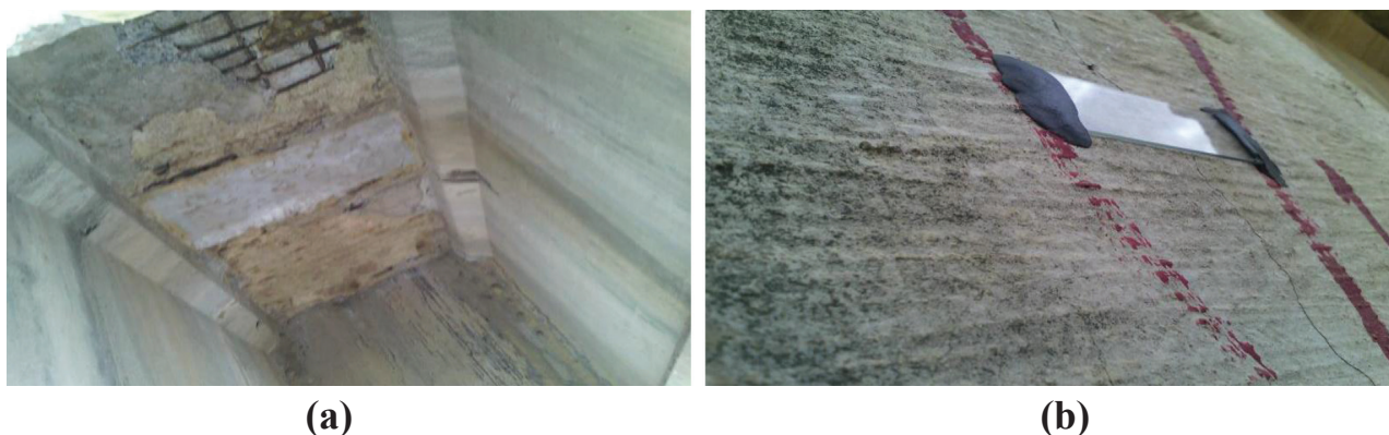
Fig 1. Deterioration of structural members of Ratlam Railway Bridge. (a) Cover delamination and corroded reinforcement exposure observed in deck slab bottom (b) Severe cracks seen in girder
