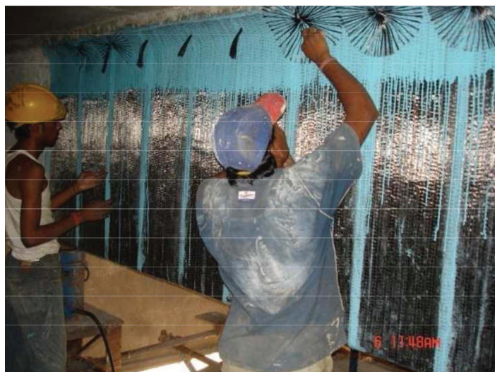
Figure 6: Enclosing the girders with carbon fiber wrapping 5
