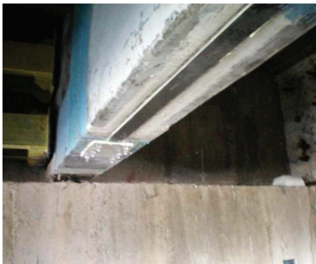
Figure 5: Prestressed laminates with anchor plates at the ends 5
