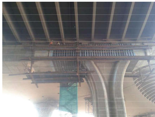
Figure 12: Strengthening of pier caps 433
