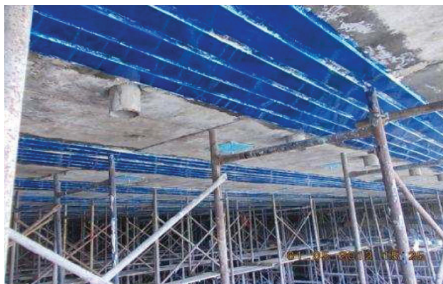
Figure 9: FRP laminates placed for flexural enhancement
