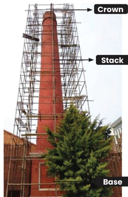
Figure 1: Important parts of chimney
