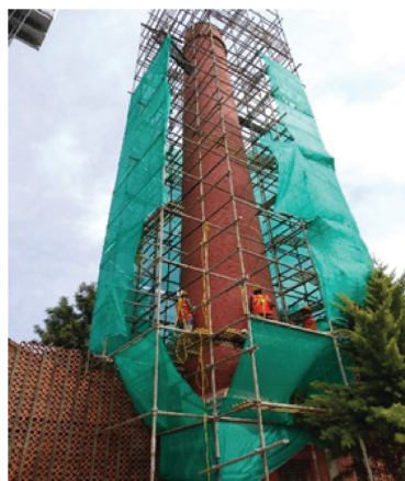
Figure 2: Erection of scaffolding around the chimney.
