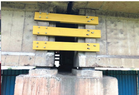
Fig.2: Steel Plate Connection between Two Girders
