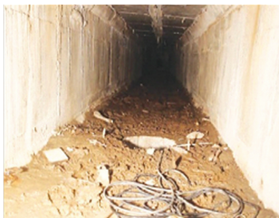
Fig. 15: Placing of Sensors
