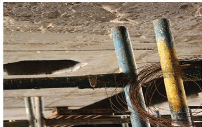
Fig.11 : Drilling of Holes
