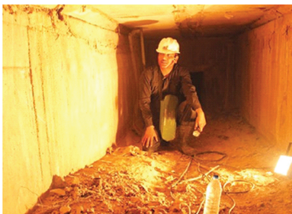
Fig.14: Inspection of Box Girder
