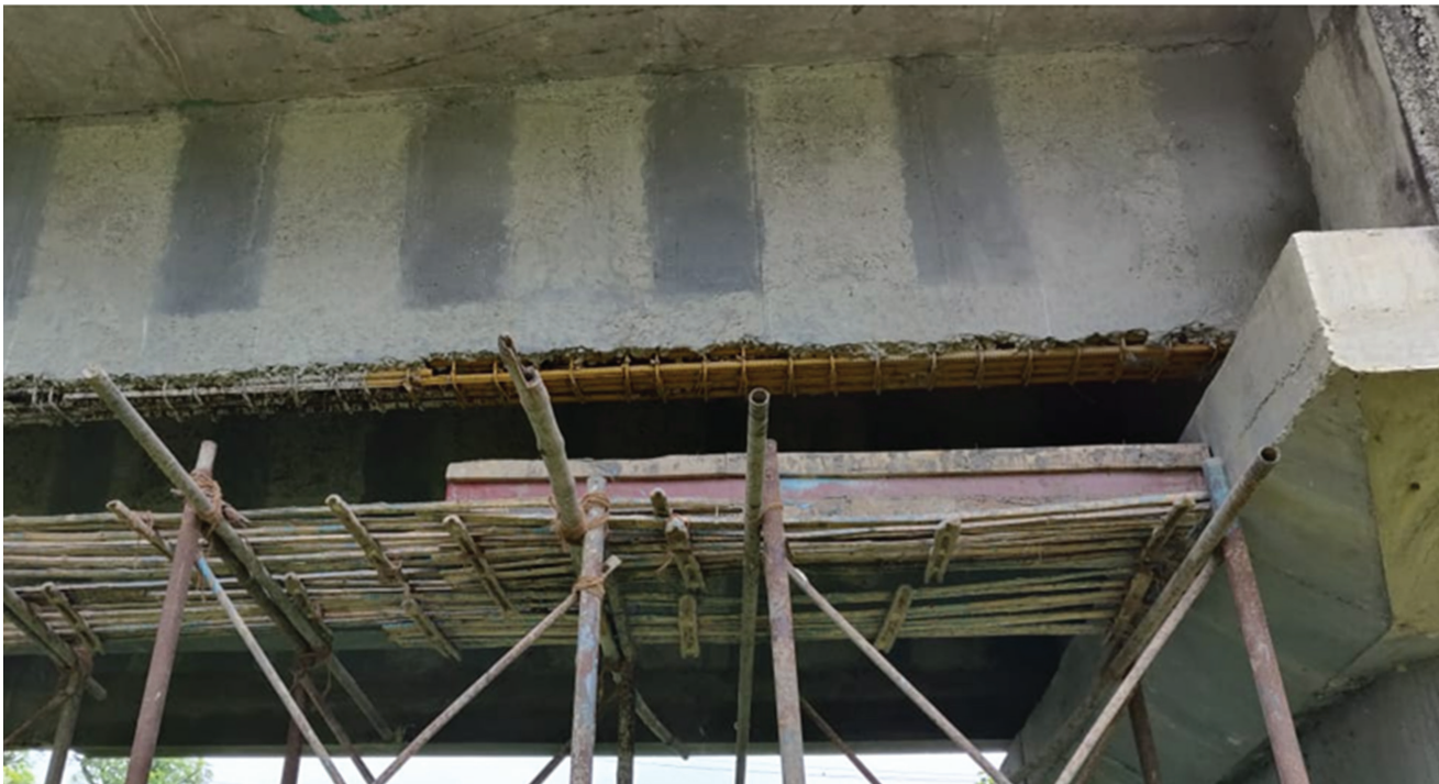
Fig. 10: Exposed Reinforcement and Anti-corrosive paint
