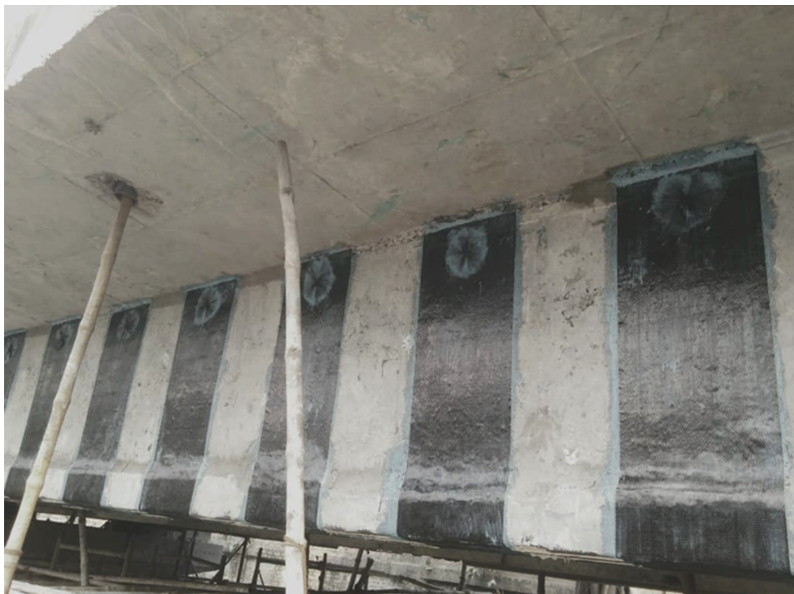
Fig. 11: RC girders Strengthened by CFRP System
