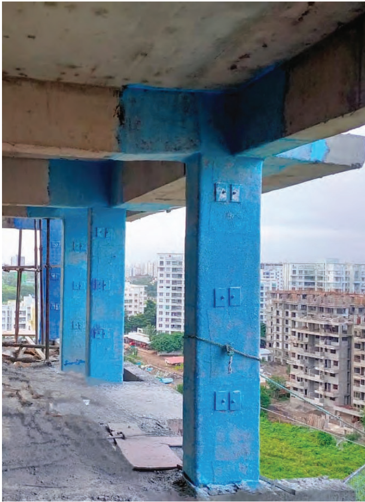
Fig: Column jacketed with prestressed CFRP system
