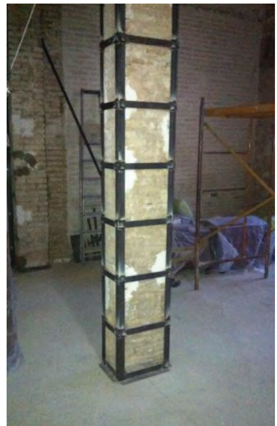
Fig: Column with steel jacketing
