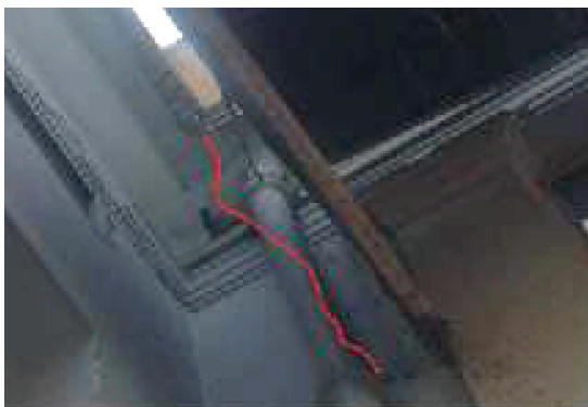
Fig. 9 Major crack developed on the first floor as seen from outside
