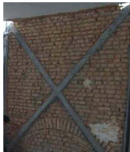
fig. 4 Diagonal Bracing of wall for strenghtening
