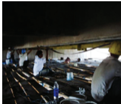
Fig. 10 Prestressing of CFRP laminates at bottom of girder [9] (Courtesy:- M/s R & M International Pvt Ltd)
