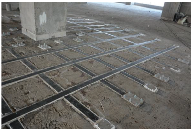
Fig.7 Application of Prestressed FRP laminates in slabs (Courtesy:- M/s R & M International Pvt Ltd)
