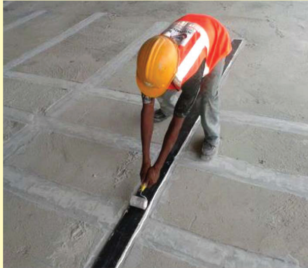
Fig.2 Application of Non prestressed FRP laminates in slabs (Courtesy:- M/s R & M International Pvt Ltd)
