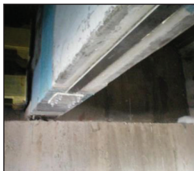
Fig. 11 Prestressed laminates with anchor plates at the ends [9] (Courtesy:- M/s R & M International Pvt Ltd)
