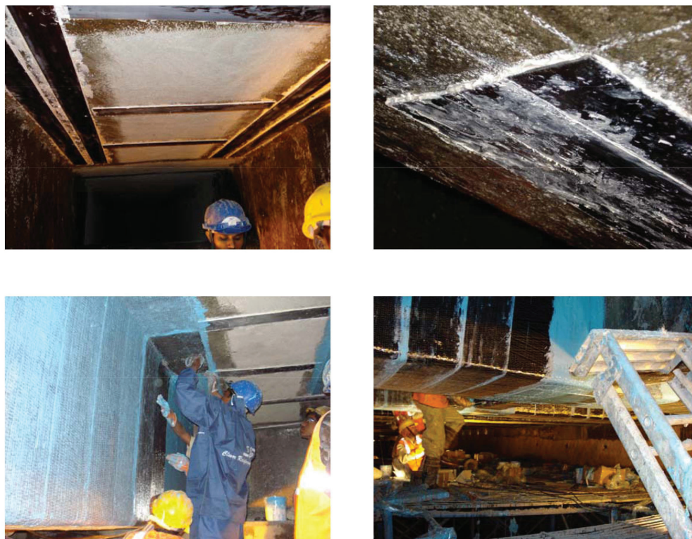
Fig. 8 Application of FRP laminates to the T-Beam at the site
