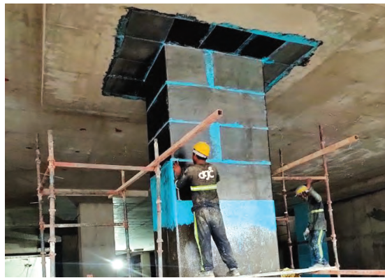
Fig. 4.5: Execution of the column strengthening with CFRP
