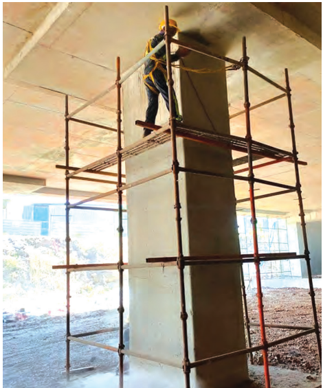
Fig. 4.2: Forming Radius at corners of the column
