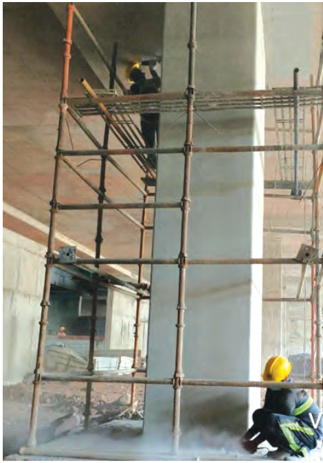
Fig. 4.1: surface preparation for CFRP strengthening
