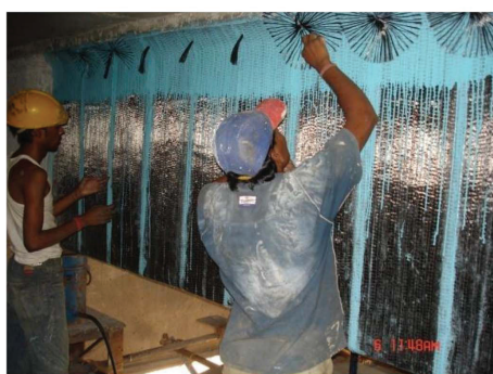
Figure 6. Enclosing the girders with Carbon Fiber Wrapping
