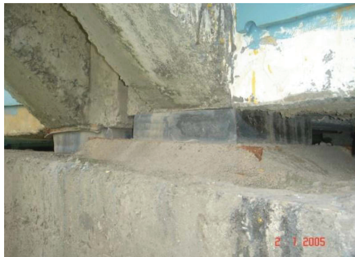
Fig. 4 Replacement of damaged Bearings with new
