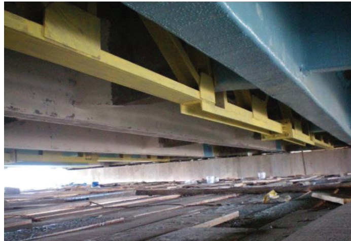
(a) Connection of Truss over Diaphragm Beam
