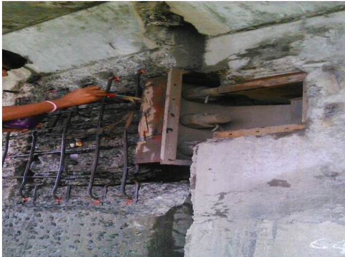
(a) Anti-rust application on exposed Reinforcement
