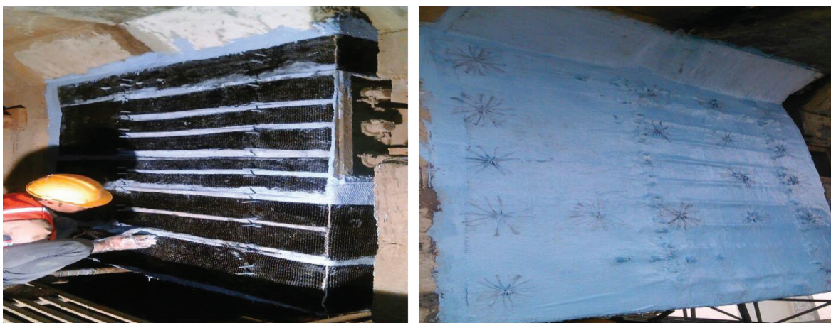
Fig 6. FRP Strengthening of Bridge's Hinge Connection Part
