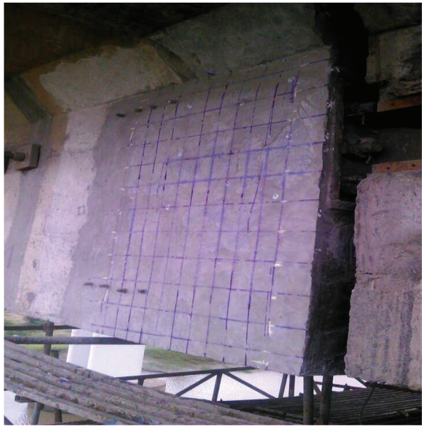
(b) Marking on New Concrete for Grooving
