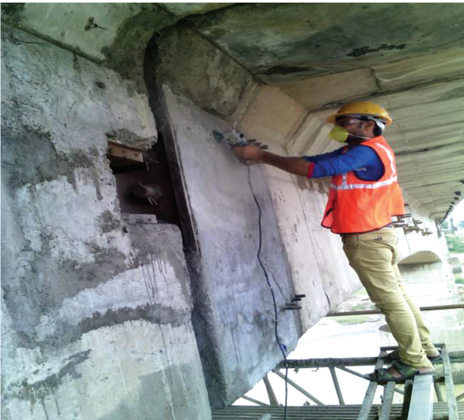
(a) Grinding of New Concrete Surface Preparation
