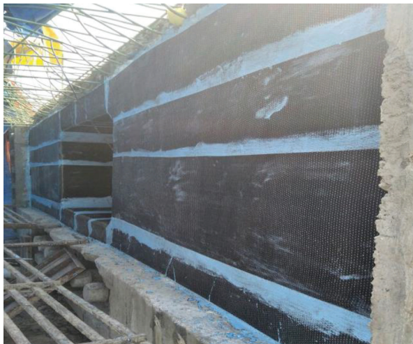
Fig 14. Application of FRP to Increase Strength
