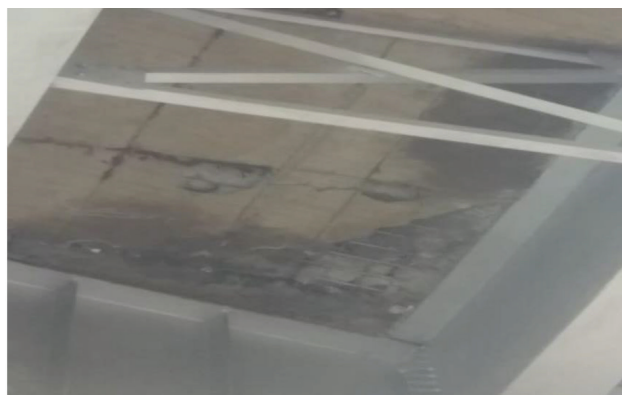
Fig 16. Bottom Side view of Distressed Deck Slab
