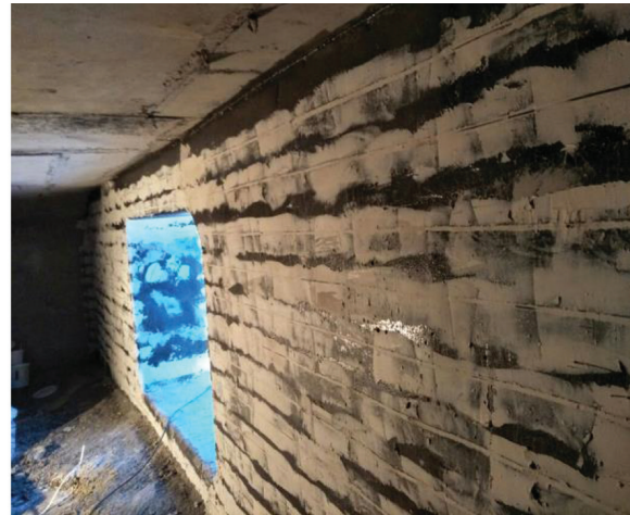
Fig 13. Laminate Fixing and Application of Putty
