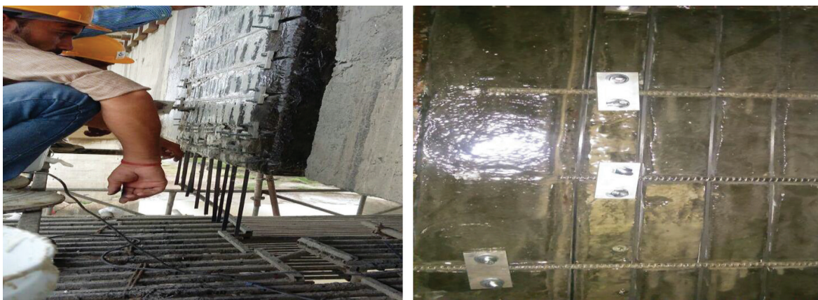
Fig 5. Fixing Additional Reinforcement on Concrete surface
