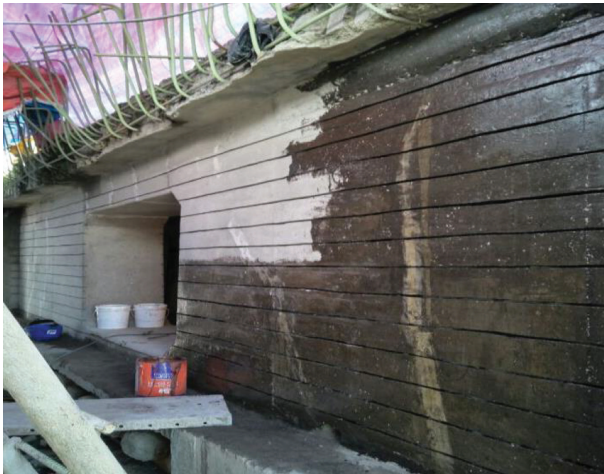
Fig 12. Grooving and Primer Application
