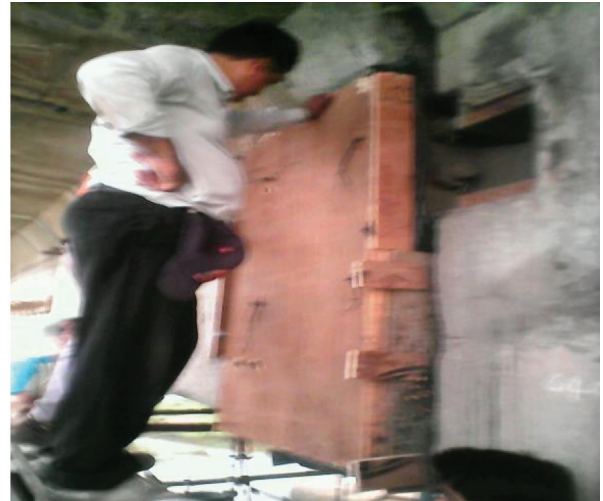
(b) Concreting of damaged part
