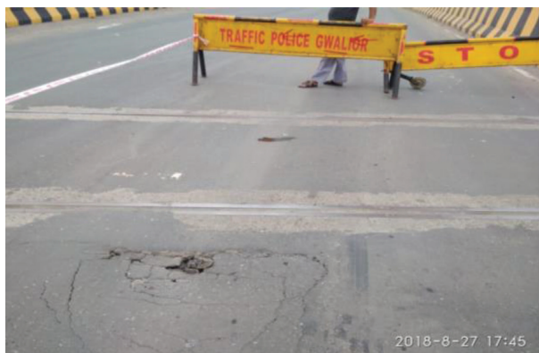
Fig 15. Distress Portion of Deck Slab
