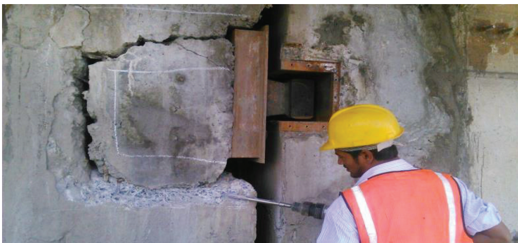
Fig 2. Failed Hinge Connection of Bharuch Bridge
