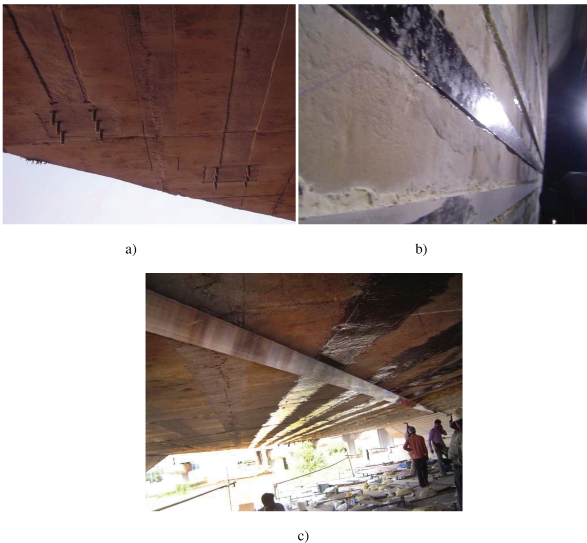
Fig 19 a) The markings and anchor bolts at place. b) Pre-Stressing of Slabs in “Cross-Traffic movement” direction with C-fiber Laminate c) Prestressing in the “Traffic movement” direction.
