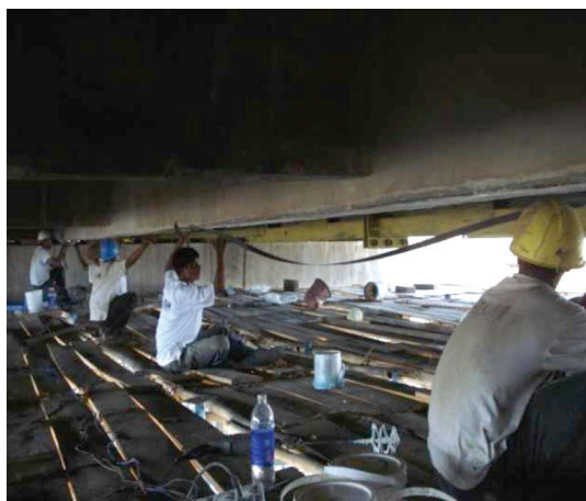
Fig 7 Pre-stressing in process and the finished laminate with anchor plates at end.
