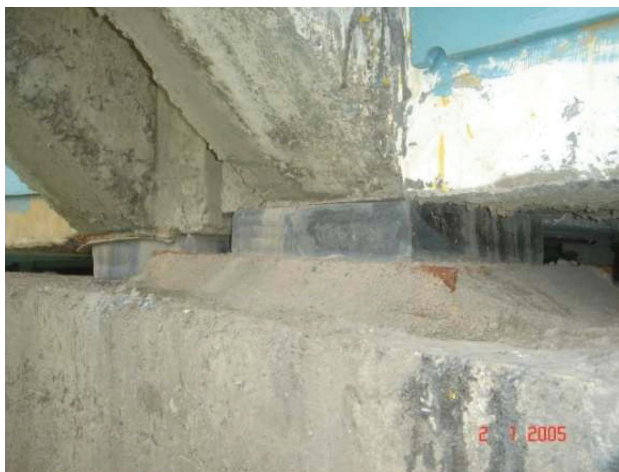
Fig. 6 Replacement of damaged Bearings with new
