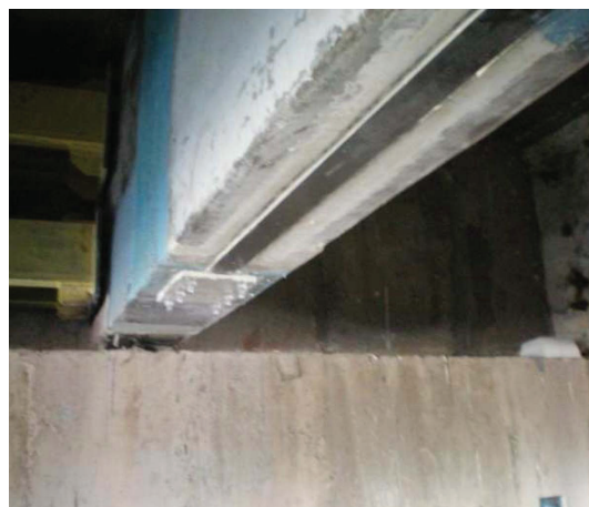
Fig 7 Pre-stressing in process and the finished laminate with anchor plates at end.
