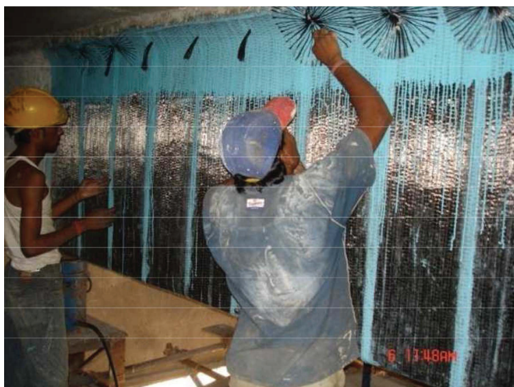
Fig 8 Enclosing the girders with Carbon Fiber Wrapping
