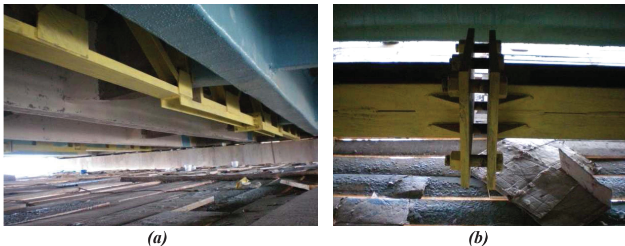
Fig. 5 (a) Connection of Truss over Diaphragm Beam and (b) Pre-stressing Mechanism in Truss During Installation of Steel Truss System
