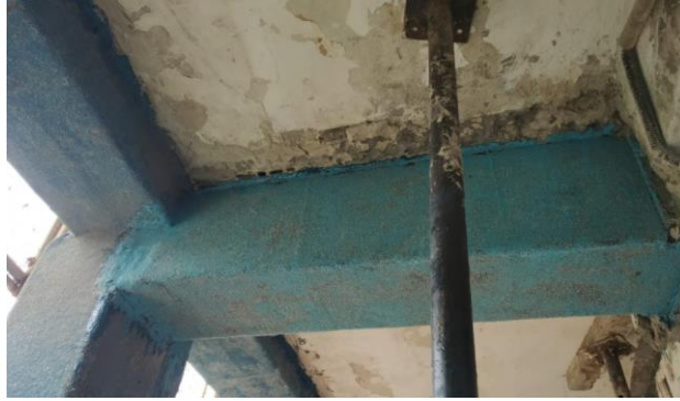
Fig 5: Beam retrofitted using R&M CFRP
