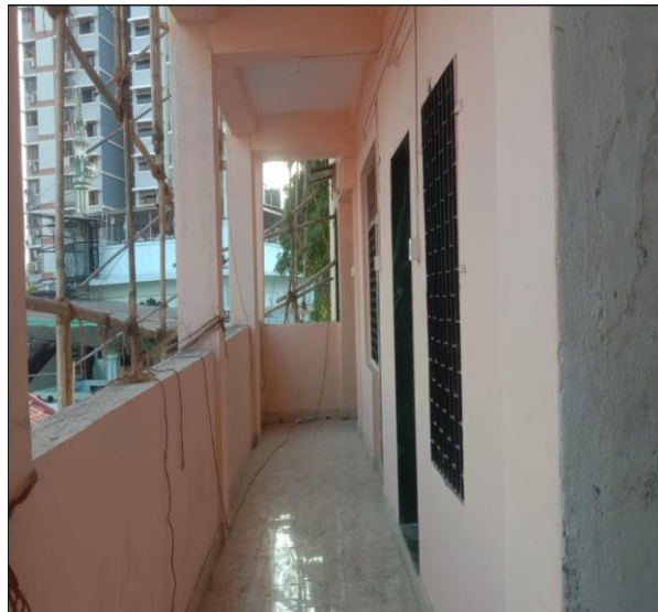
Fig 8: Building Interiors after rehabilitation
