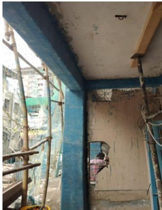
Fig 6: R&M CFRP wrapping on columns
