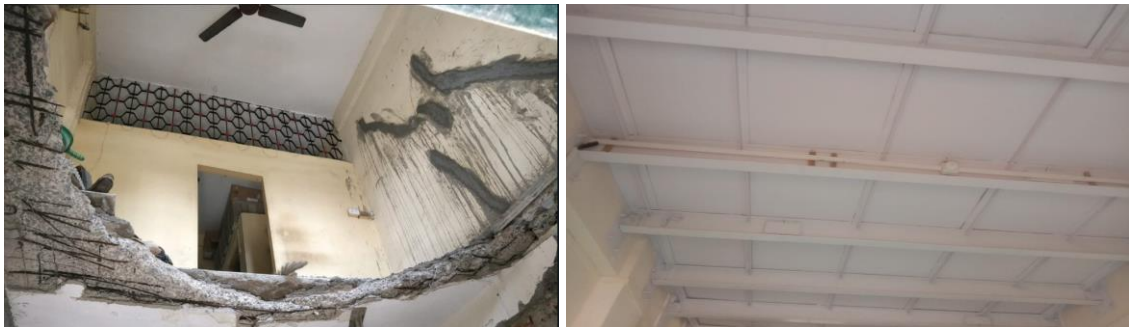
Fig 4: Recasting of slab with Aerocon Sandwich Panels
