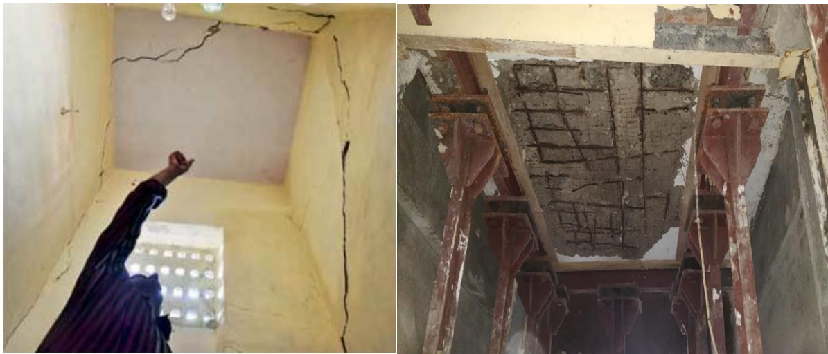
Fig 1: Building image before rehabilitation
