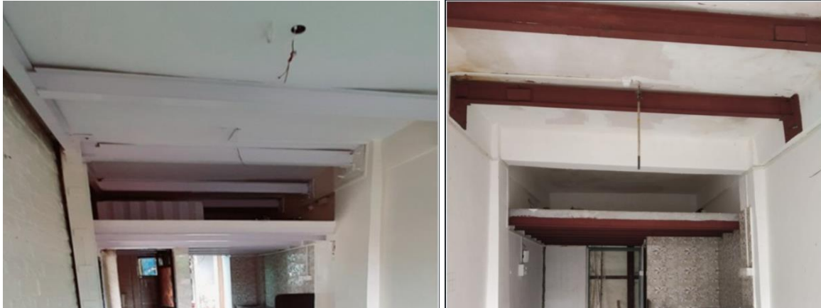
Fig 2: Introduction of steel beam to arrest slab deflection
