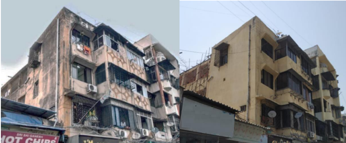
Fig 9: Building before and after rehabilitation
