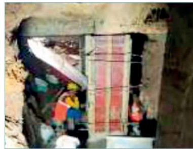
Fig. 5: Column Strengthening
