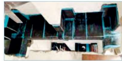
Fig. 9: Beam Strengthening with CFRP Wrapping
