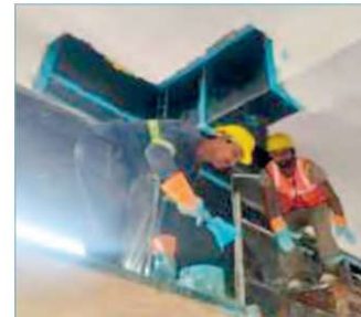
Fig. 10: Column-beam Junction Confinement with CFRP
