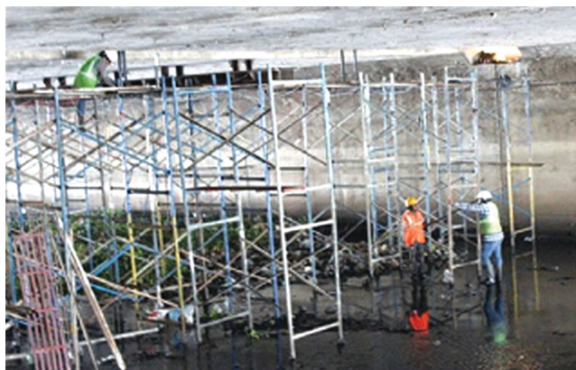
Fig.10 : Erection of Scaffolding
