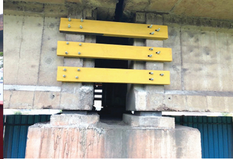
Fig.2: Steel Plate Connection between Two Girders
