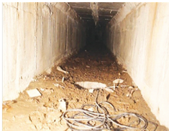
Fig. 15: Placing of Sensors
