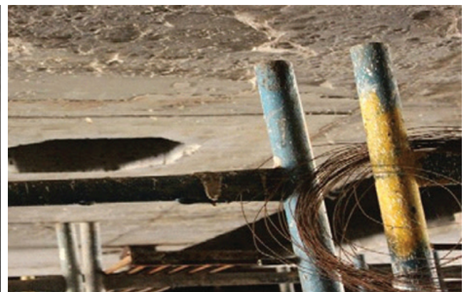
Fig.11 : Drilling of Holes
