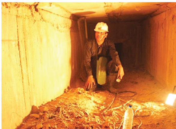
Fig.14: Inspection of Box Girder
