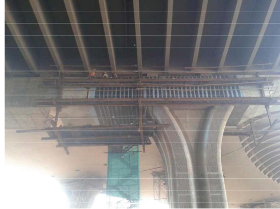
Figure 12: Strengthening of pier caps 433
