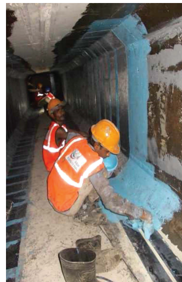
Figure 10: CFRP fiber wrapping being done for shear strengthening of girders
