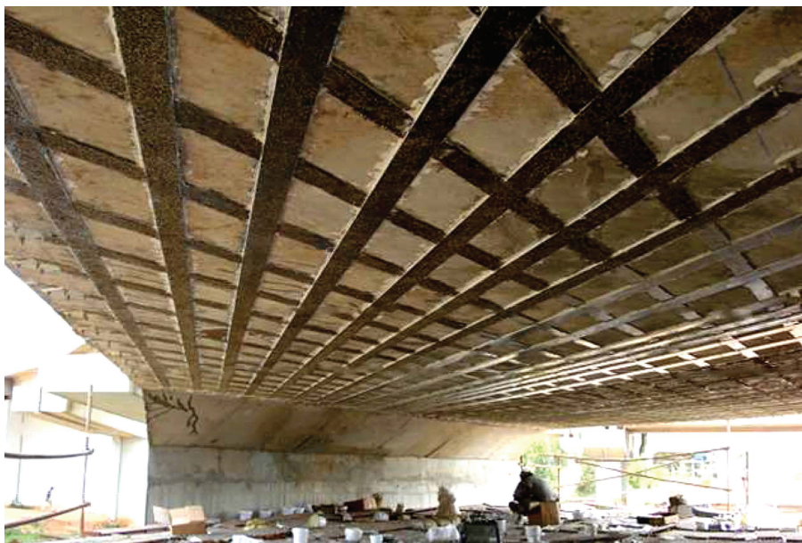
Figure 2: Strengthening of Skew slab using FRP laminates
