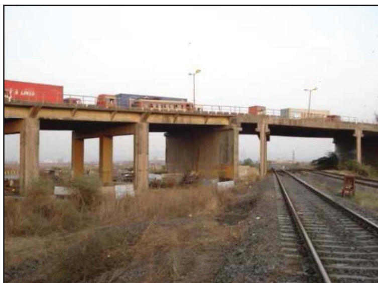
Figure 3: Rail Over Bridge (ROB) at Karal junction of JNPT 5
