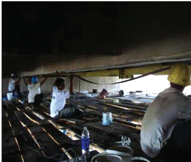
Figure 4: Prestressing in process for the girder s
