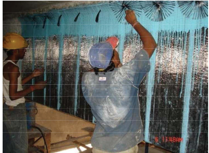
Figure 6: Enclosing the girders with carbon fiber wrapping 5
