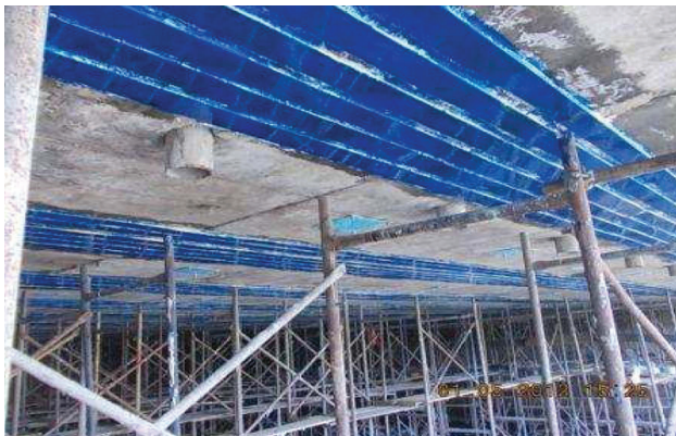
Figure 9: FRP laminates placed for flexural enhancement
