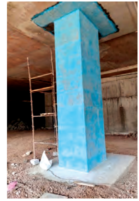
Fig. 4.6: Finished Column after the top coating sand sprinkling
