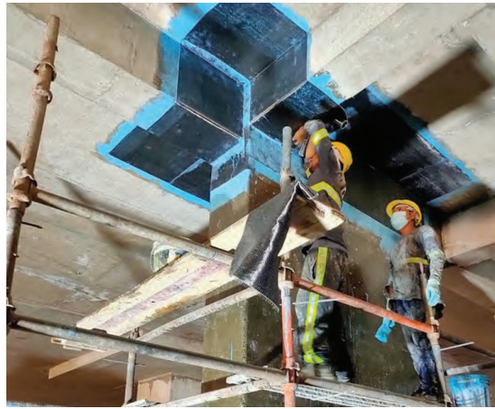
Fig. 4.4: beam-column junction confining with CFRP
