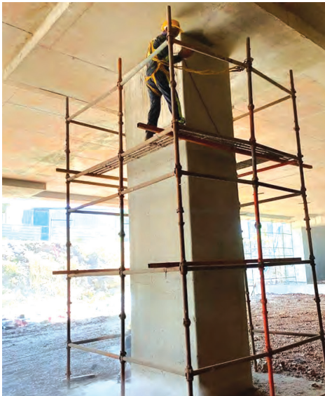
Fig. 4.2: Forming Radius at corners of the column
