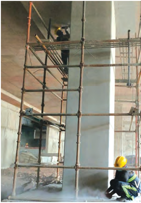
Fig. 4.1: surface preparation for CFRP strengthening
