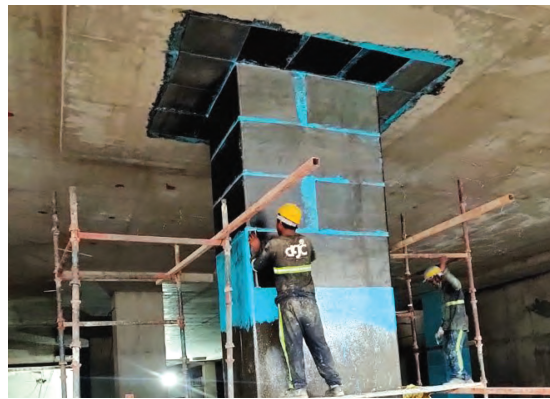
Fig. 4.5: Execution of the column strengthening with CFRP
