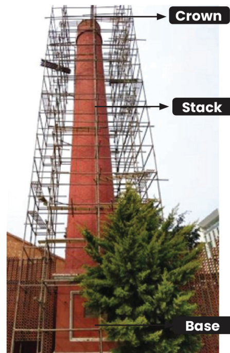
Figure 1: Important parts of chimney
