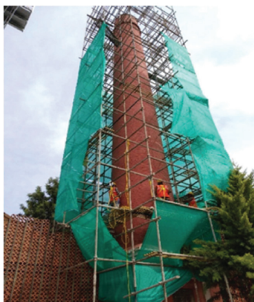
Figure 2: Erection of scaffolding around the chimney.
