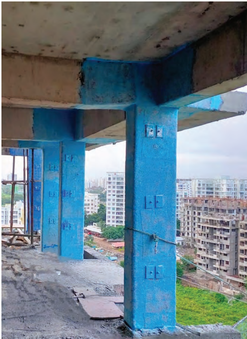
Fig: Column jacketed with prestressed CFRP system
