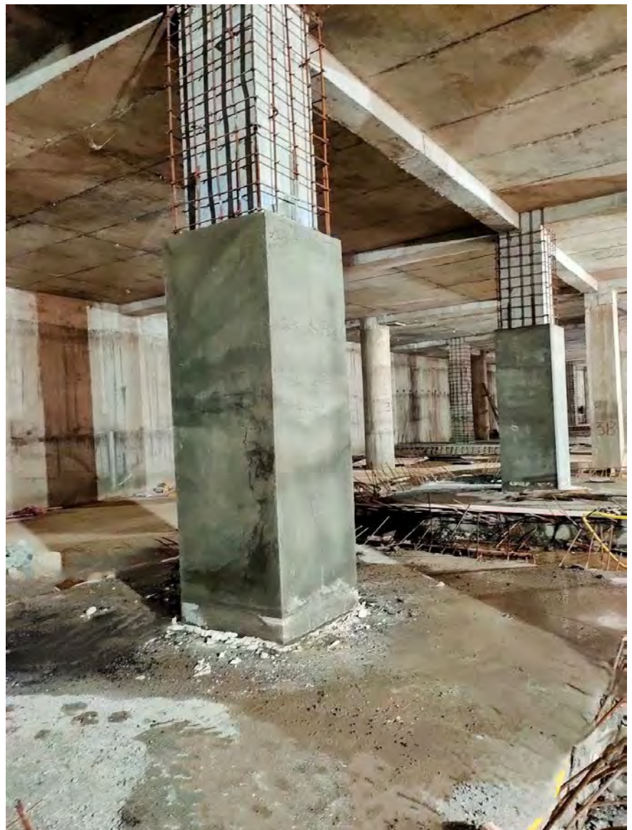
Fig 3.1.2: Geometry and reinforcement details of RC-jacketed column
