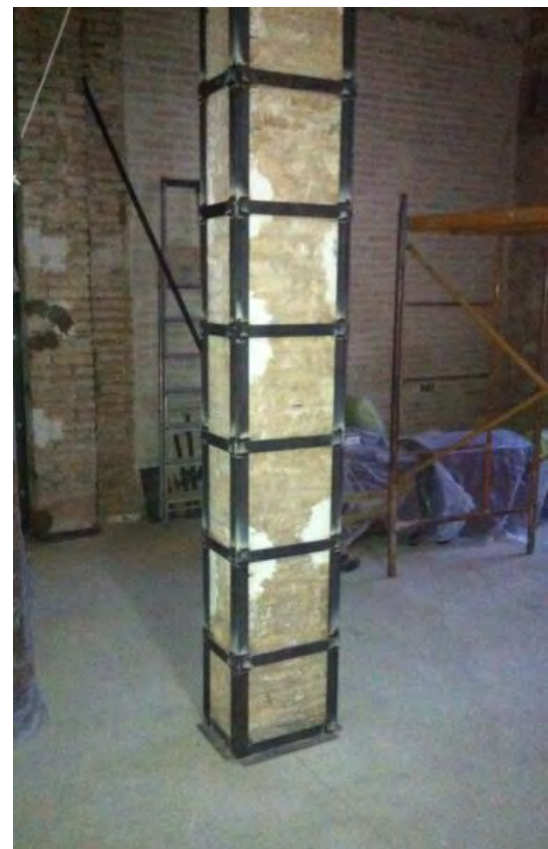
Fig: Column with steel jacketing
