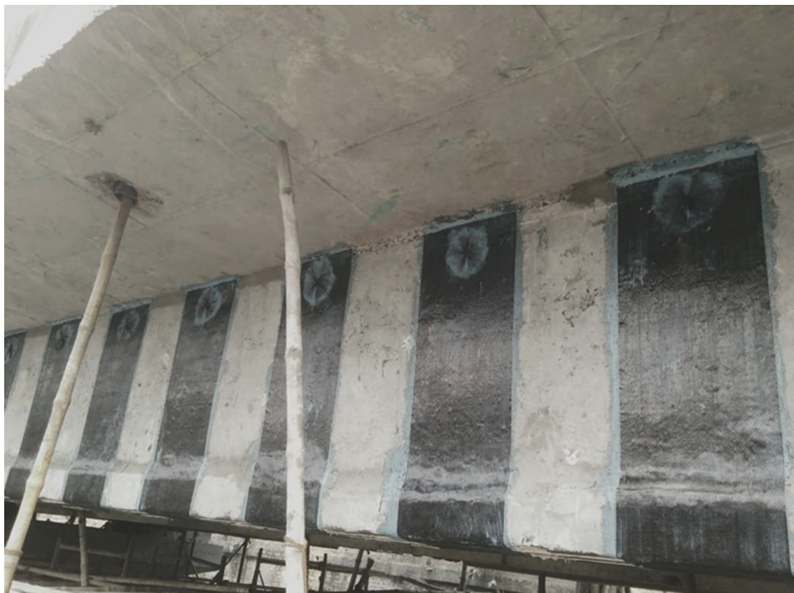
Fig. 11: RC girders Strengthened by CFRP System
