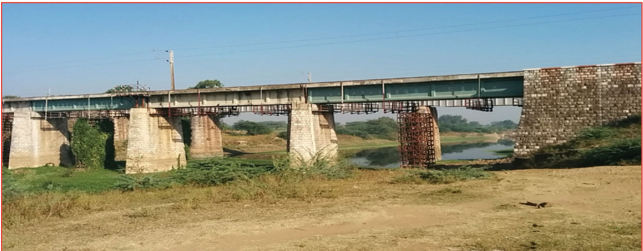
Fig. 1 Site view of raw bridge no. 114
