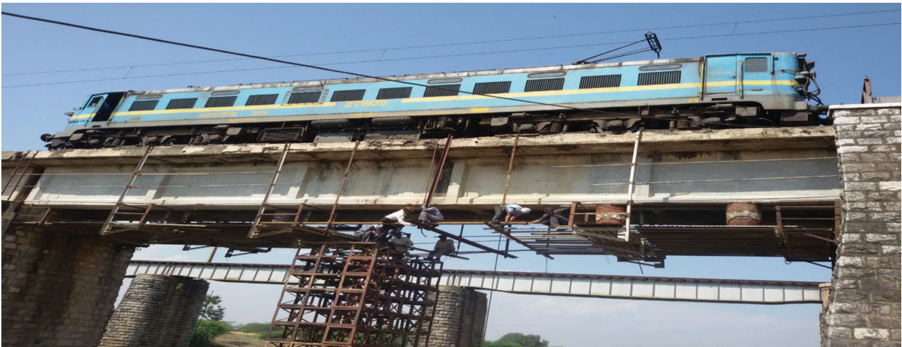
Fig. 6 Load applied on the bridge using Wagon 7 and sensors at site
