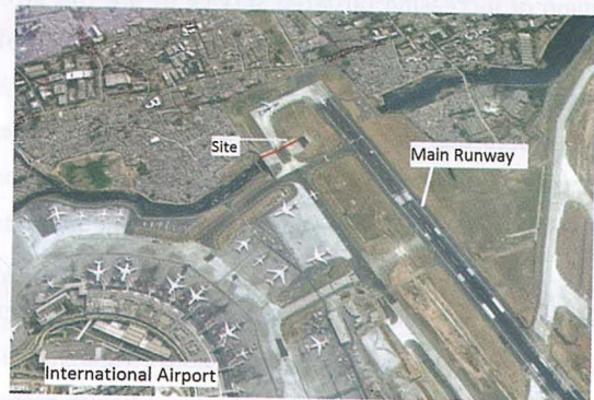
Fig.2: Position of Mithi River Bridge below the Runway
