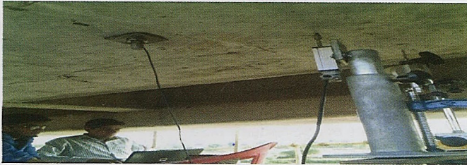
Fig.2: Structural Health Monitoring of Ratlam Railway Bridge with Help of Sensor
