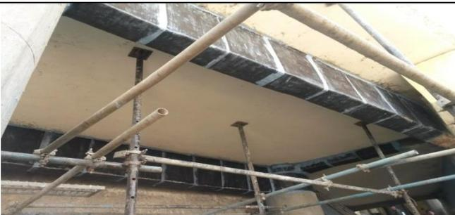
A photograph showing a concrete beam being wrapped with carbon fiber. The beam is supported by a network of steel reinforcement bars. The carbon fiber is applied in a spiral pattern around the beam, and the surface is smooth. The background shows a construction site with wooden formwork and other structural elements. | Carbon fiber wrapping on beam ( 430 GSM) |
