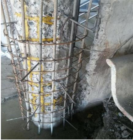
A photograph showing a cylindrical reinforcement cage for a concrete column. The cage is made of steel bars (rebar) arranged in a spiral pattern. The cage is positioned inside a concrete structure, and some yellow markings are visible on the bars.                                                                           | Additional new reinforcement             |
