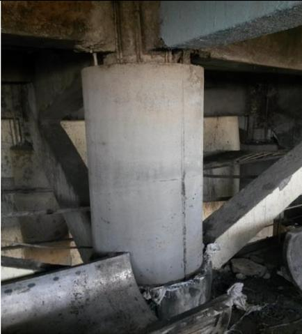
A photograph showing a concrete column being repaired or reinforced. The column is surrounded by a network of steel reinforcement bars. The repair area is filled with a light-colored concrete mixture, likely micro-concrete, which is being applied to the existing structure.                                                | Micro-concreting of column.              |
