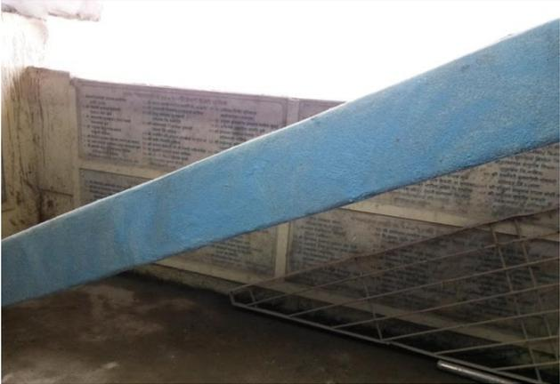
A photograph showing a concrete beam being repaired. The beam is covered with a blue epoxy putty. The putty is applied in a thick layer, and the surface is smooth. The background shows a construction site with wooden formwork and other structural elements.                                                               | Epoxy putty application on beam          |
