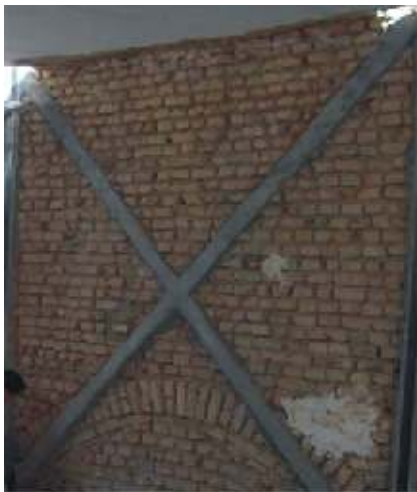
Fig 4: Diagonal Bracing of wall for strengthening
