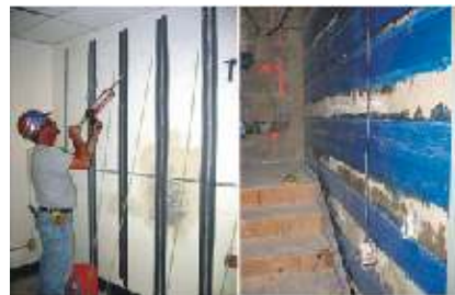
Fig 1. Flexure and shear strengthening of the walls using FRP Composites
